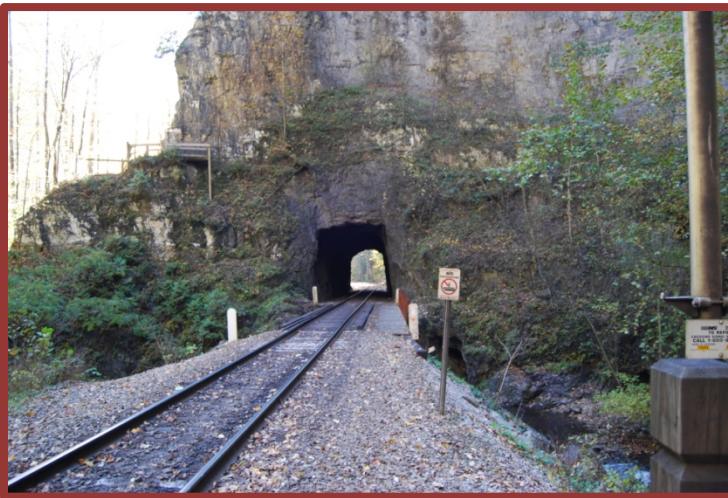
A bored tunnel just to the south of the south portal
